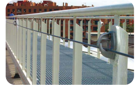
Detail of PS14 mounting plates on metal structure
