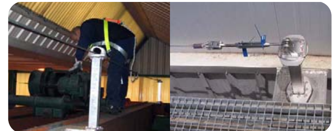
Detail of mounting column post on overhead crane
